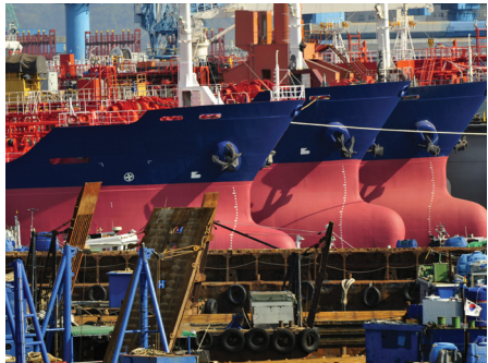
Dockside Loading Equipment
