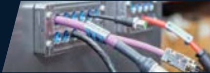
Switchgear & Cabinet Construction
