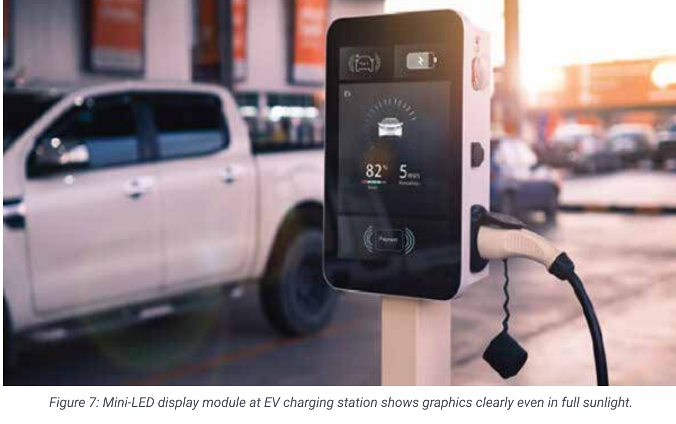
Figure 7: Mini-LED display module at EV charging station shows graphics clearly even in full sunlight.
