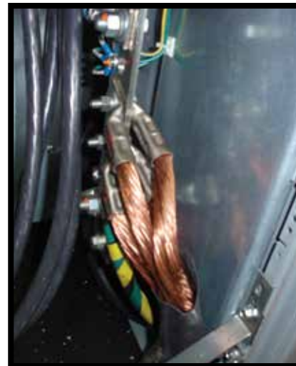
Figure 1. Termination for parallel ground connections on drive.
