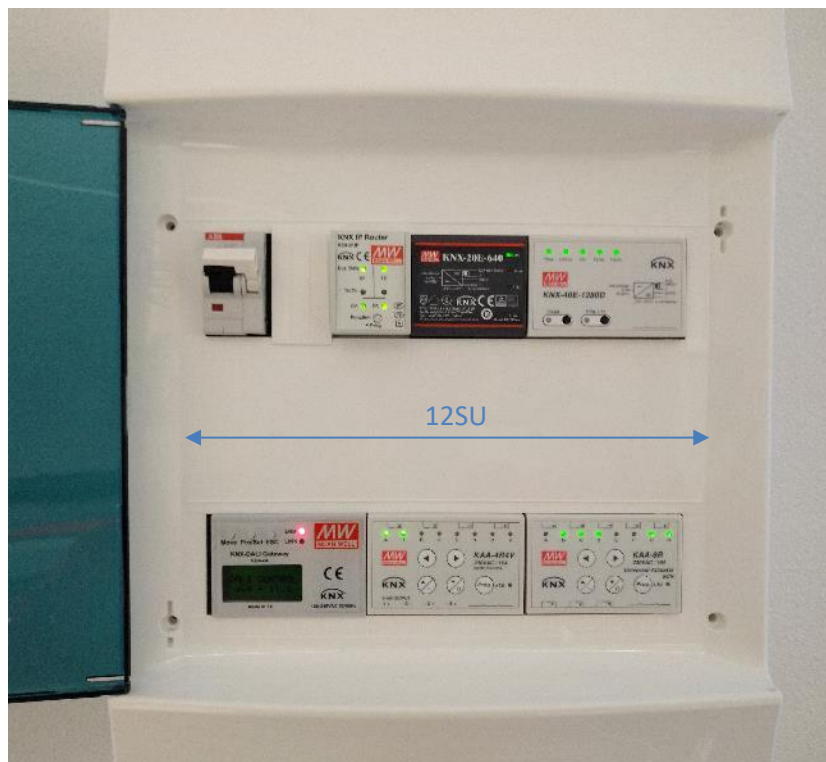
Figure 4 A common 2 rows 12 SU distribution board cabinet with installation of circuit breaker and KNX devices
