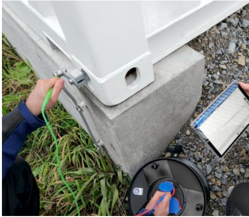
Everyday life in the installation of systems: The quality of the grounding system is measured
